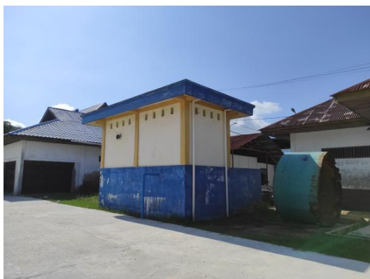
Gambar 13. Sumur bor Figure 13. Boreholes Sumber: Hasil penelitian
