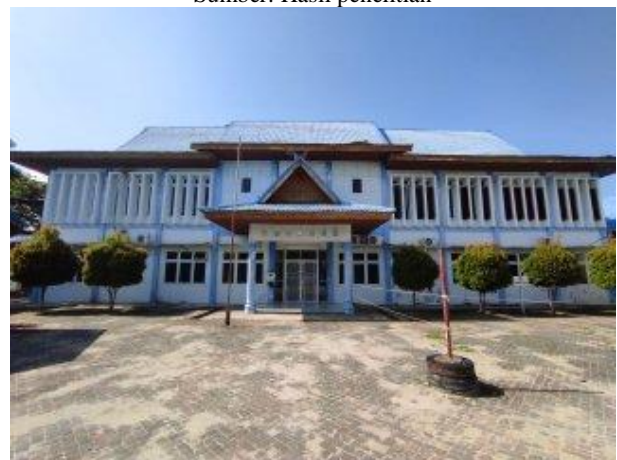
Gambar 7. Kantor Laboratorium PMHP Figure 7. PMHP Laboratory Office Sumber: Hasil penelitian
