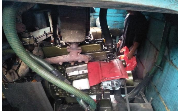
Gambar 1. Kamar mesin KM. Semi Jaya Figure 1. Engine room of KM Semi Jaya
