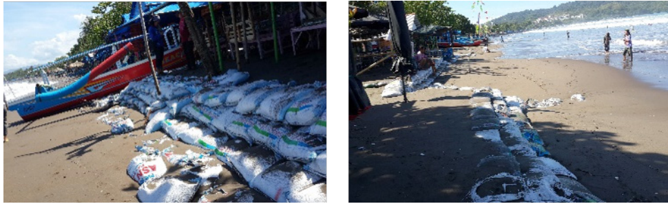
Figure 6. Sand bags that are arranged to protect the coastline wave erosion in western coast of Pangandaran.
